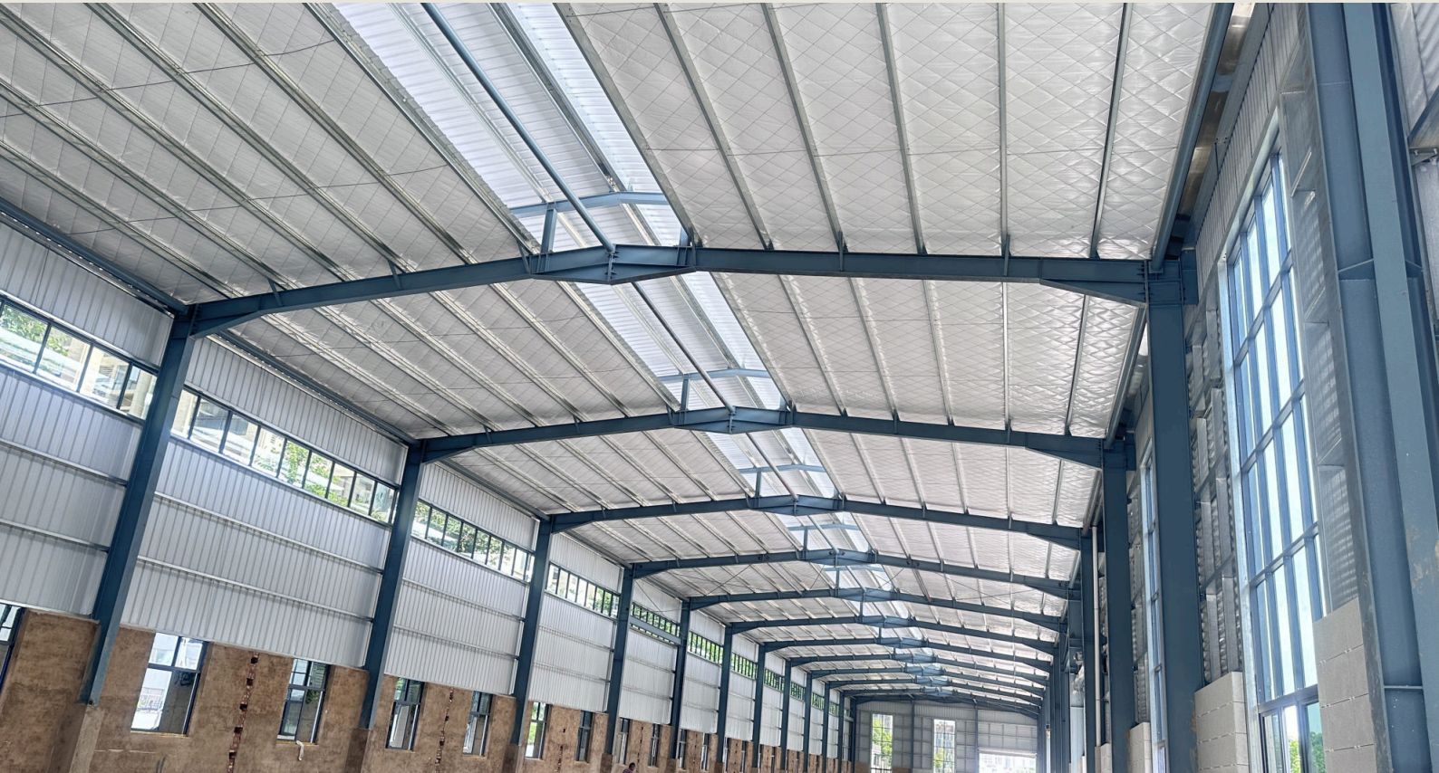
Covered-market building / site photograph
