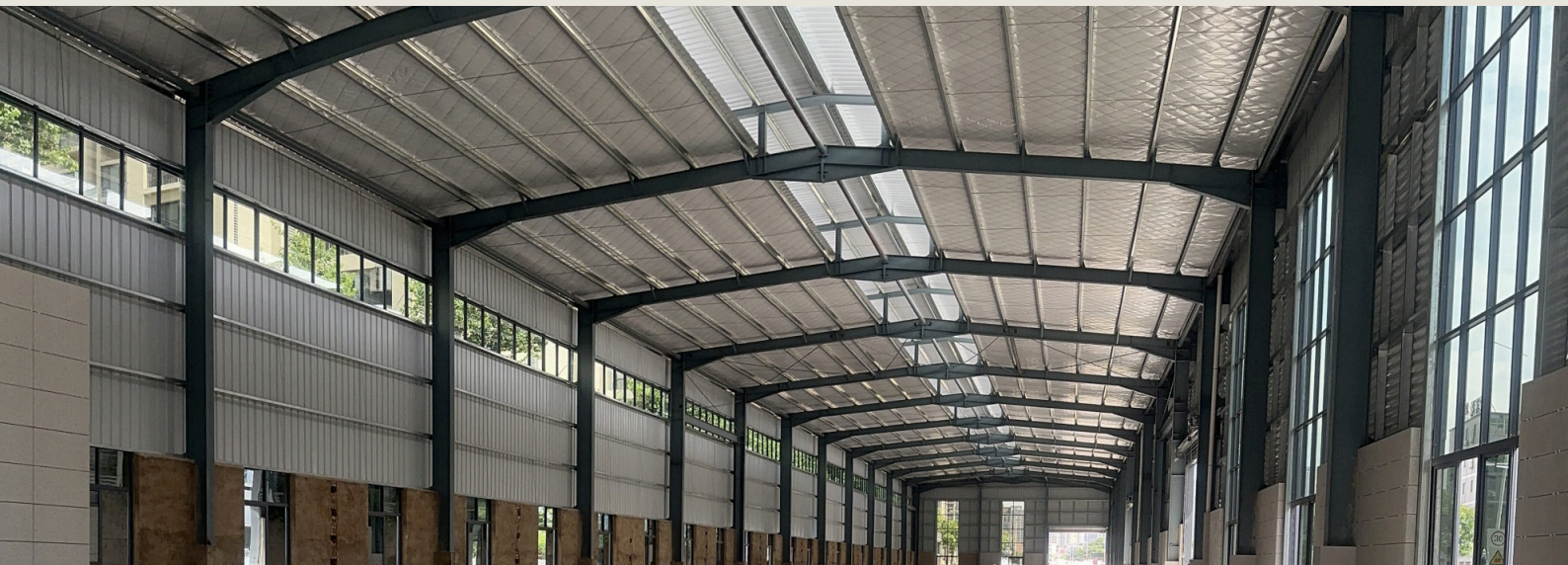
Roof and frame detail / same project
